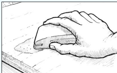
Figure 23 Sand cured fairing compound to desired contour.
